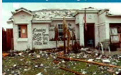
Level 3 - Major damage; uninhabitable
