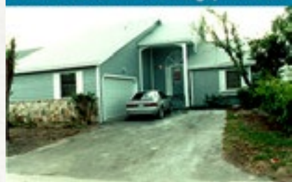
Level 2 - Major damage; habitable
